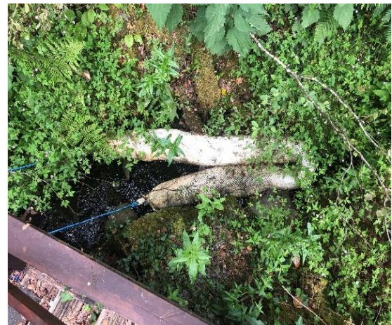
Photo Collection 6: Northern Outlet Pipe (NOP) discharge into unnamed stream with oil skimmer, north of the site NGR - SH 68917 38507
